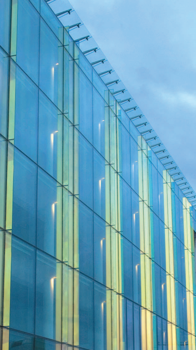
Different viewing angles and varying weather conditions result in a change of the color impression of NARIMA® color effects glass. Grand Canal Square 1, Dublin, Architect: Duffy Mitchell O'Donoghue (DMO'D)
