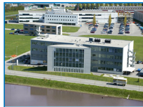
SCHOTT’s site in Yverdon – the new center of excellence for optical components
