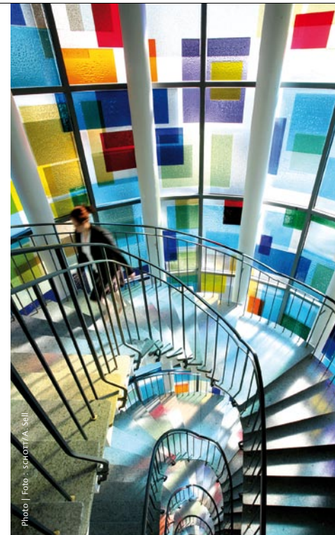
Thin-film modules were integrated into this staircase designed with Artista® colored glass.
