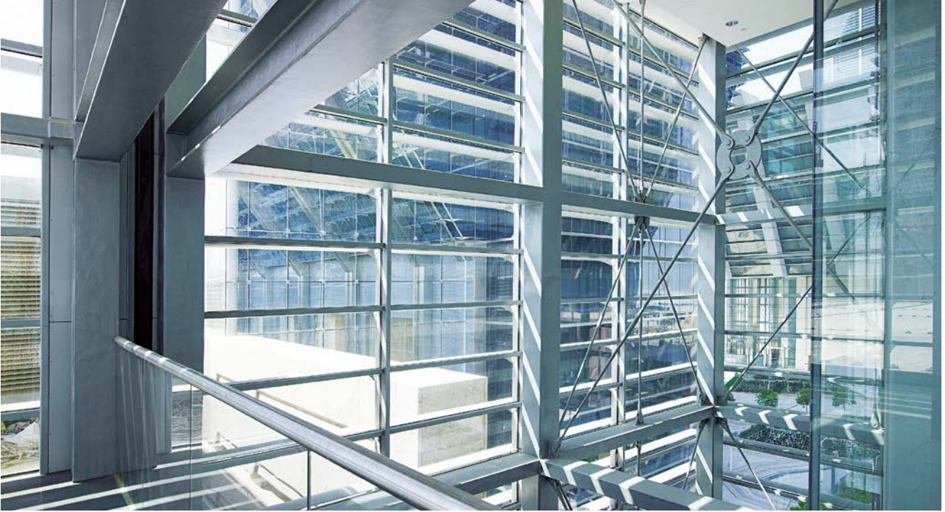
Anti-Reflective Glass for the facade of the Abu Dhabi Financial Car Park
