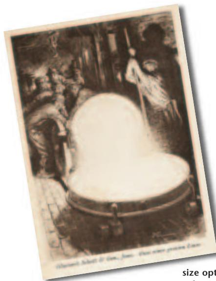
Using the “Jena casting process” Otto Schott produced large
