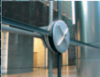
The round metal medallions attached to the corners of the glass panes are the joints for the network of steel cables and also stabilize the glass facade.
