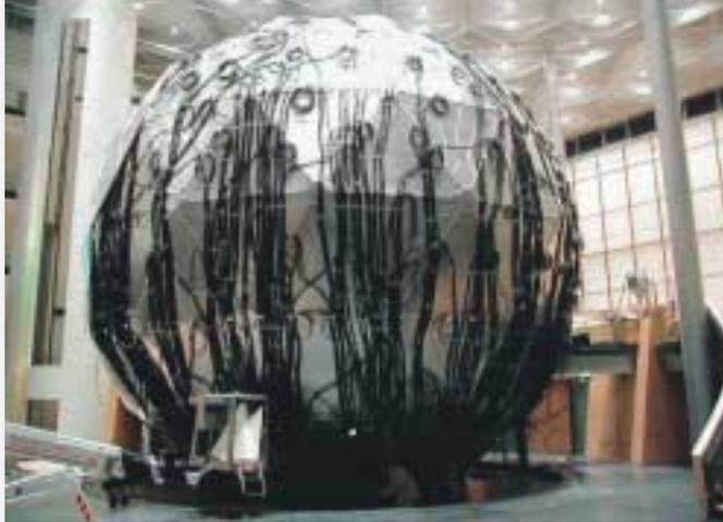
Intricate inner workings: the individual light panels of the illuminated "Kugelhaus" are supplied with light from 20 kilometers of light conducting cables.
