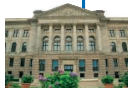
In the Bundesrat Building in Berlin, lighting elements with "Conturax" profile rods enhance stylish surroundings with pleasant lighting.
